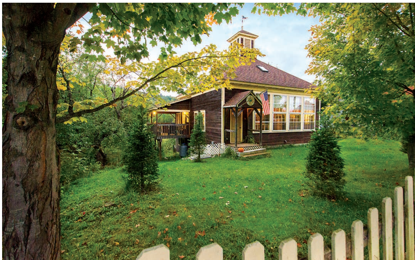
During the initial restoration, Jerry removed the old roofing, replaced it with new shingles, and renovated the existing cupola. Inside, and reachable through a wood-framed ceiling hatch (complete with stained-glass depictions of Vermont's birds made by Tim Gustafson Byrne), is a bell. You can open the hatch and ring the bell by pulling ropes on the main floor.
